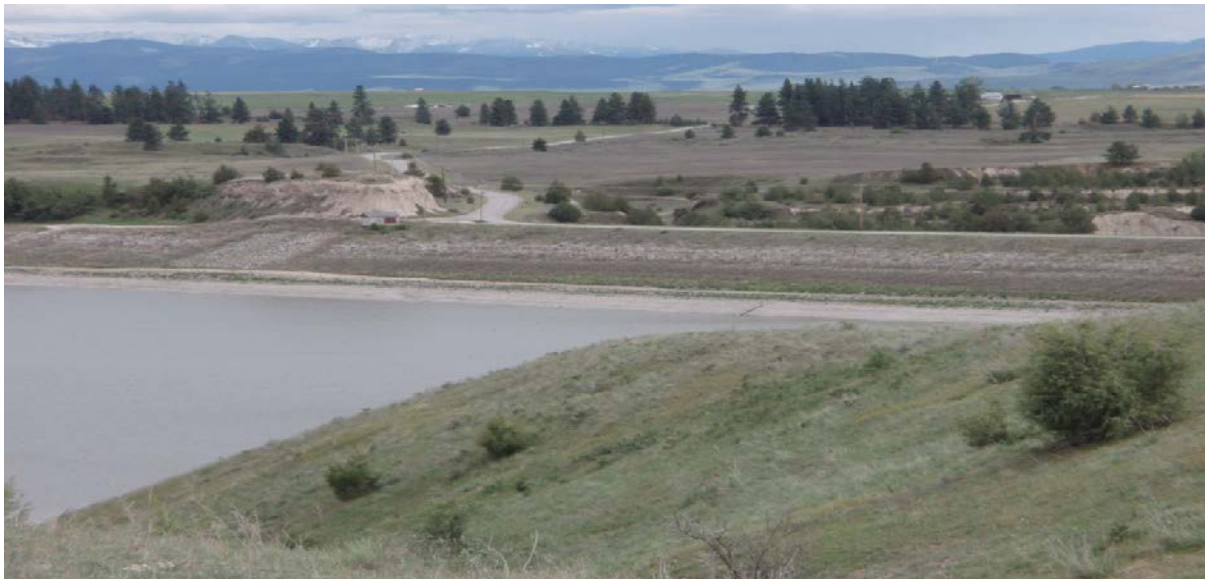
Crow Dam, Flathead Indian Reservation, Montana
