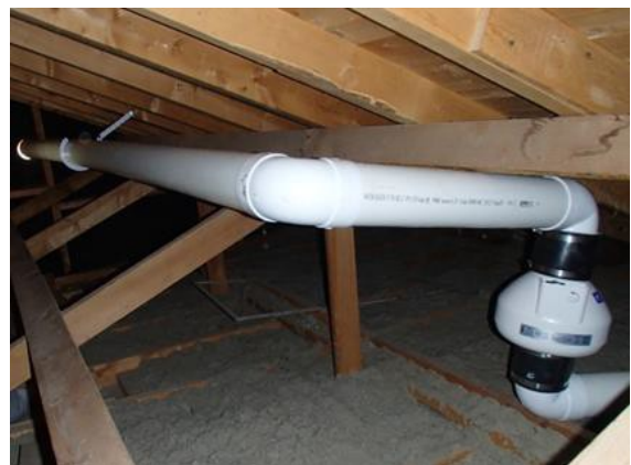
Radon Exhaust Fan Installed at Blackfeet Dormitory Quarters Units
