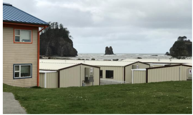
Quileute Tribal School Portable Classrooms
