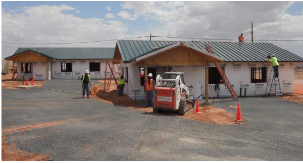
Moencopi Quarters under Construction
