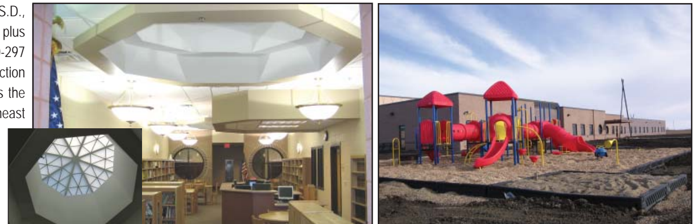
The Enemy Swim Day School features skylights and chandeliers throughout the one-story building which sits amid lakes and rolling hills with pastures full of roaming buffalo.
