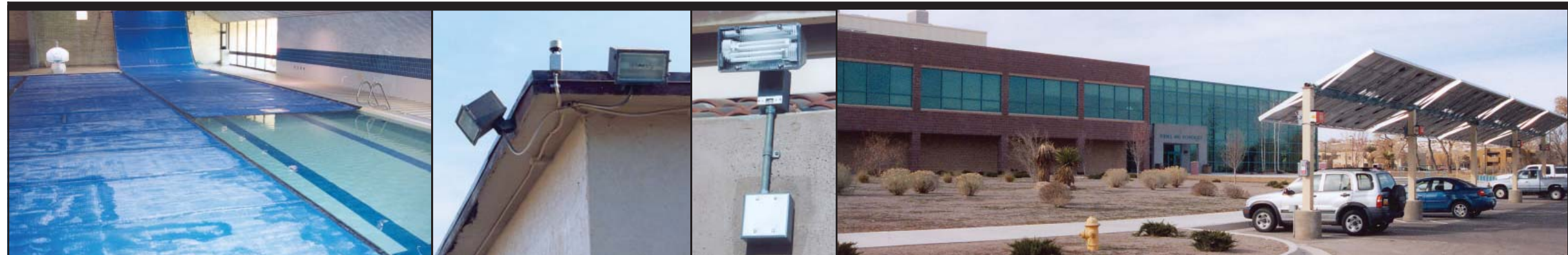
(1) When not in use, the pool at Sherman Indian High School (SIHS) is covered to retain the water's heat. (2) A daylight sensor between two lights on SIHS campus automatically turns the lights on or off. (3) Outdoor lighting at SIHS now features lamps which use 90 percent less energy, yet provide equivalent lighting as high-energy-use floodlights. (4) The Science and Technology Building parking lot at the Southwestern Indian Polytechnic Institute features solar panels which track the sun.
