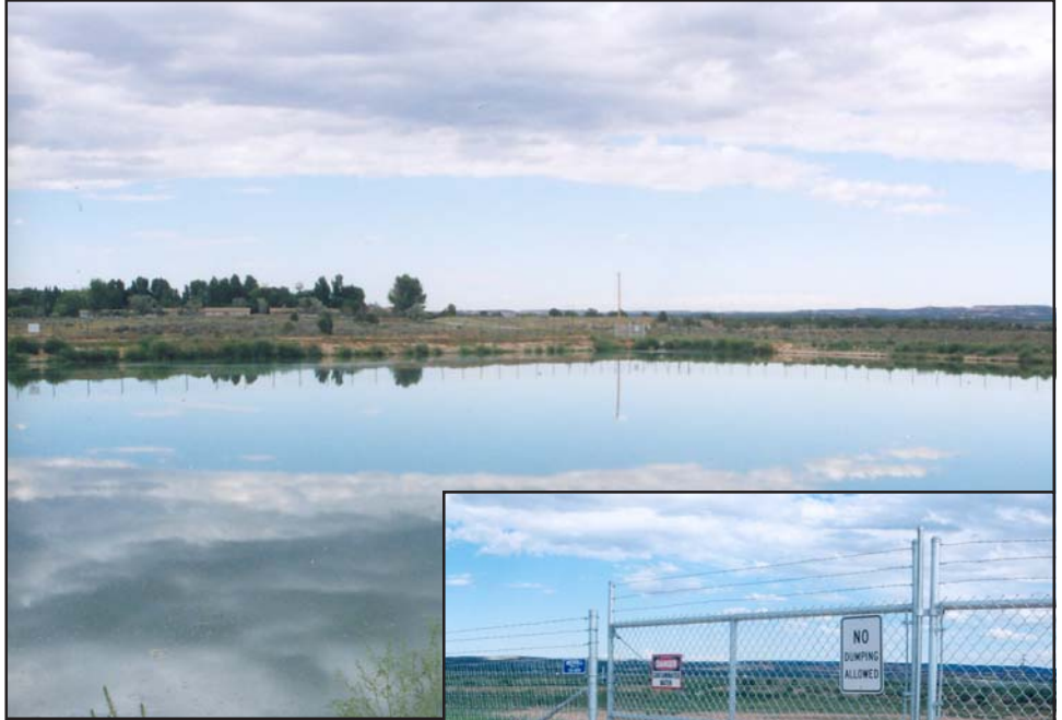
Shonto Preparatory School's six sewage ponds were upgraded this year with the removal of sludge, the renovation of dikes and the installation of replacement fencing and piping, all part of the Navajo Region's sewage lagoon improvements.
