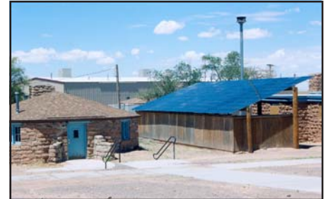
Seba Dalkai's solar panel generated electricity for the old school.
