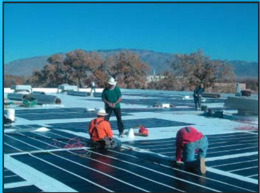
SIPI's roof meets Cool Roof Rating Standards.
