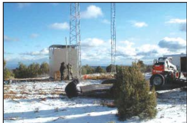
Tower renovation work gets underway in New Mexico.
