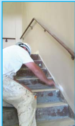
The interior surfaces are painted with low volatile organic compound (VOC) paint to reduce the amount of paint-based gases leeching into the air.
