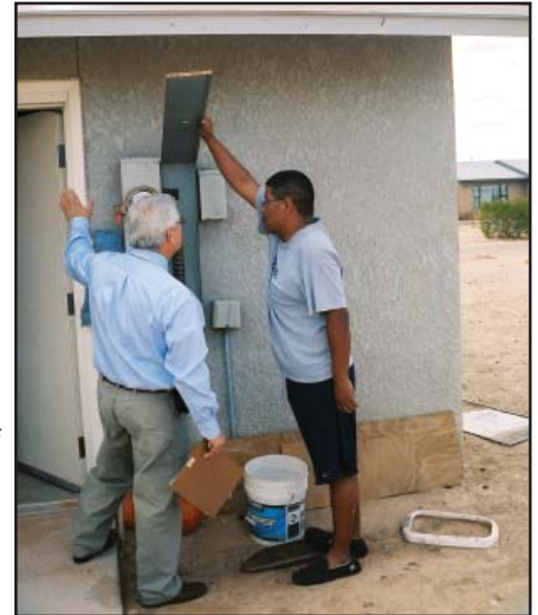
Employee housing assessment inspector Michael Morrison (left) inspects the electric connections of a home at Tohono O'odham High School in Arizona. Helping is renter Carl Antone.
