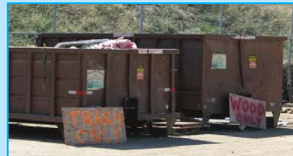
About 85 percent of construction waste is being collected in separate bins to be recycled into post-consumer products.
