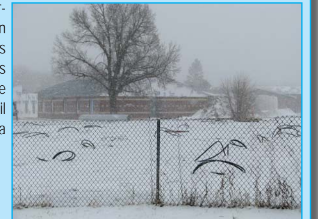
Tubes linking the ground source heat pump wells next to the new Pine Ridge School dormitory in South Dakota emerge through a spring 2009 snow.
