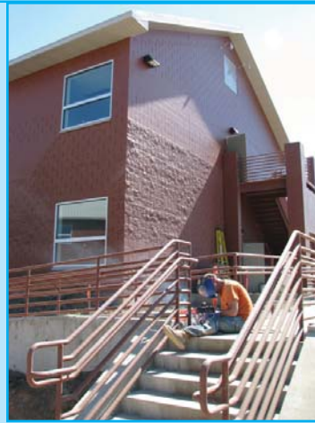
A worker welds the handrails (right) leading to a side entrance of the new Chemawa dormitory (below).
