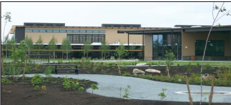
Rain from the Muckleshoot roofs flows into this and other school rain gardens.
