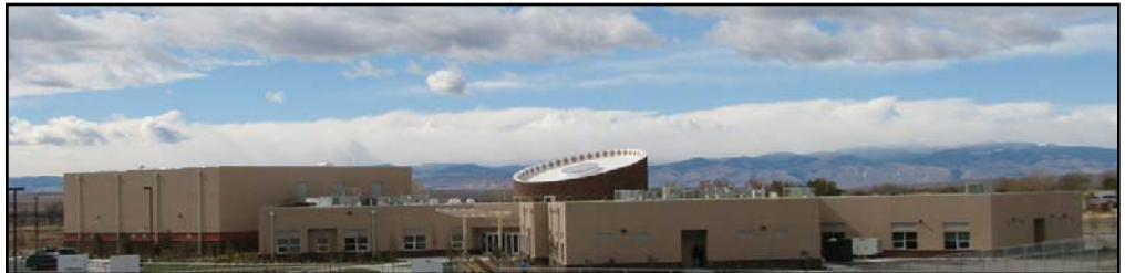
Once housed in a 1950’s-era mission building, St. Stephens’ new high school opened in September 2010.
