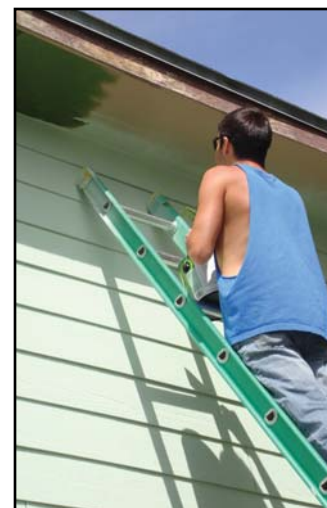
Nicholas Barnaby, a Spokane Agency OJT worker, paints a federal facility.
