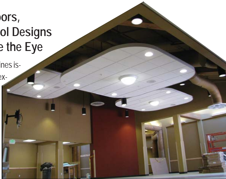
The cafeteria ceiling at Ojo Encino Day School in New Mexico.
