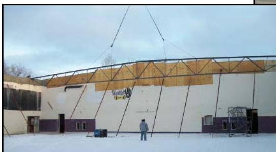
The Shonto Preparatory School gym is readied (right) this summer for student use following a January 2010 roof collapse (left) due to a winter storm that dumped 24 inches of snow on the Arizona school.
