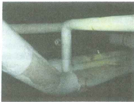
New pipe insulation
