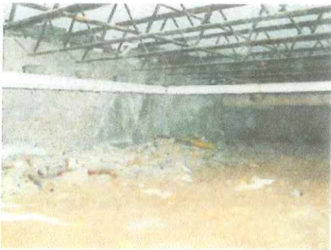
Crawl space view
