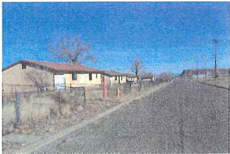
Pavement and Sidewalks
