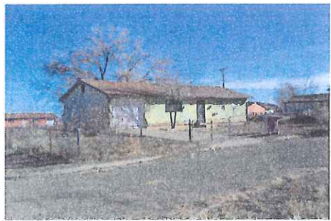
Pavement and Sidewalks
