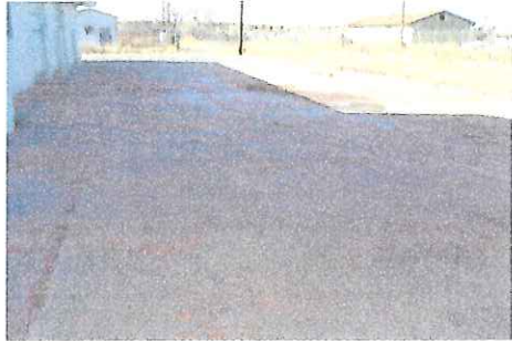
Pavement and Sidewalks
