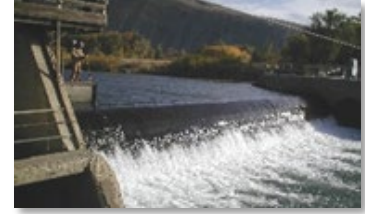
Wapato Diversion Dam on the Yakima River
